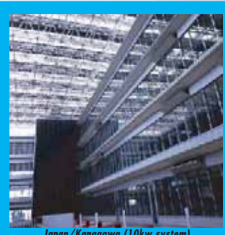
Japan/Kanagawa (10kw system)
