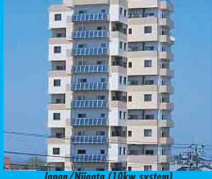
Japan/Niigata (10kw system)
