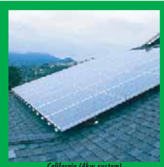
California (4kw system)
