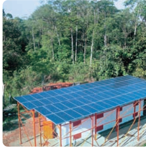
Remote telecom base station
